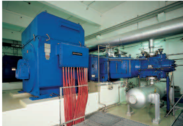
Piston-type gas compressor, driven by a converter-fed motor, 1,900 kW, 2 x 920 V, 14 poles, IP55 with top-mounted water/air heat exchanger IM B3
