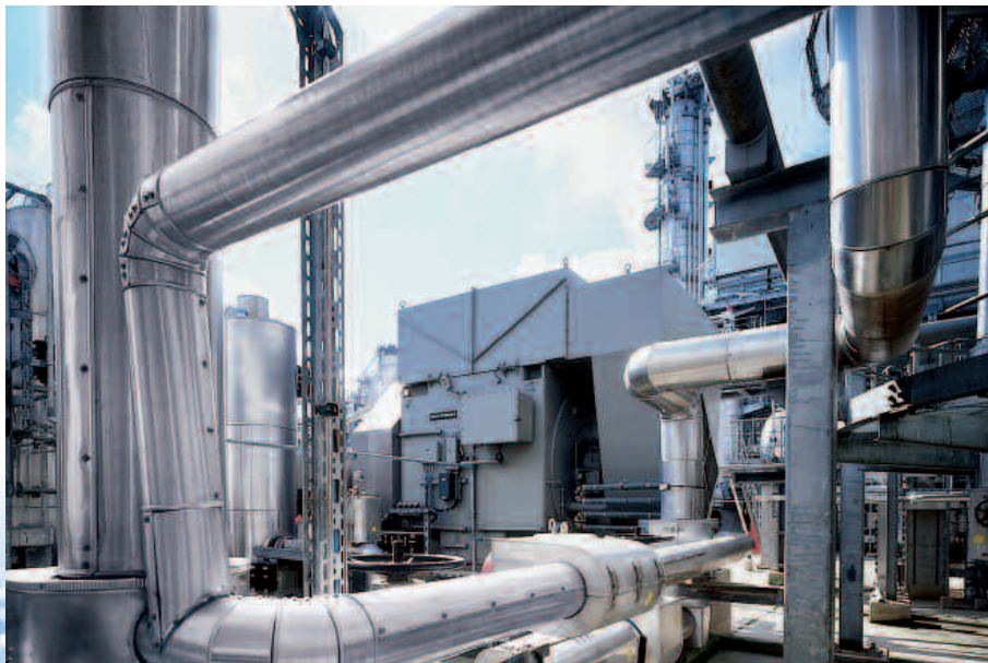
Piston-type gas compressor in an oil refinery, 3,500 kW, 6 kV, 18 poles, non sparking Ex nA II, IP55 with top mounted tube-type air/air heat exchanger, IM 1205
